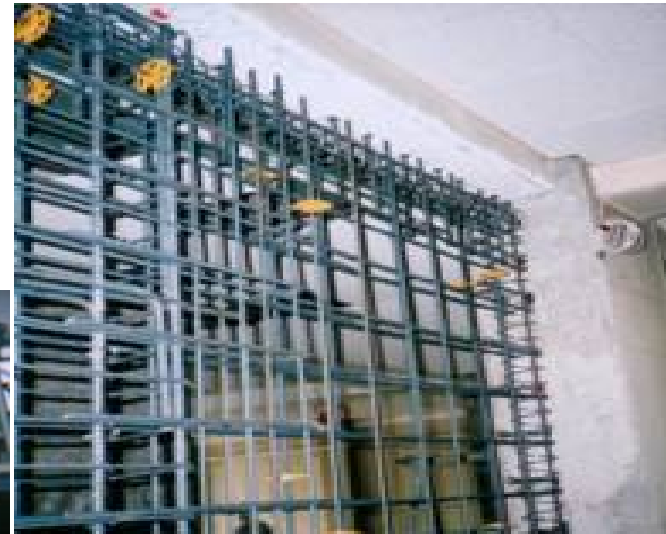
Reinforced concrete wall
