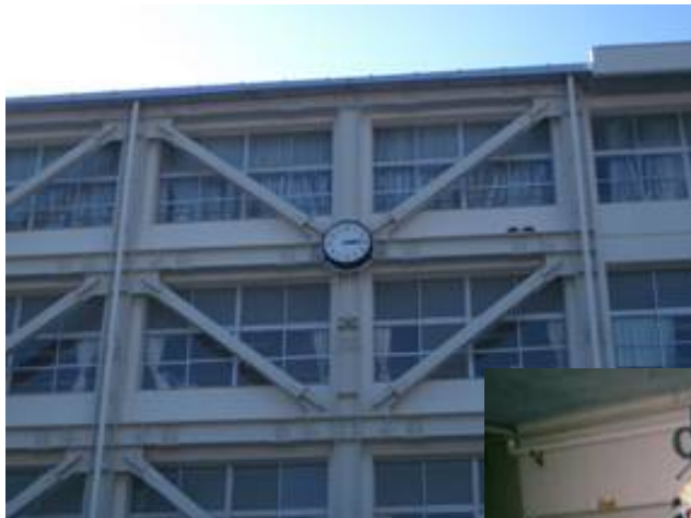
Steel frame brace
